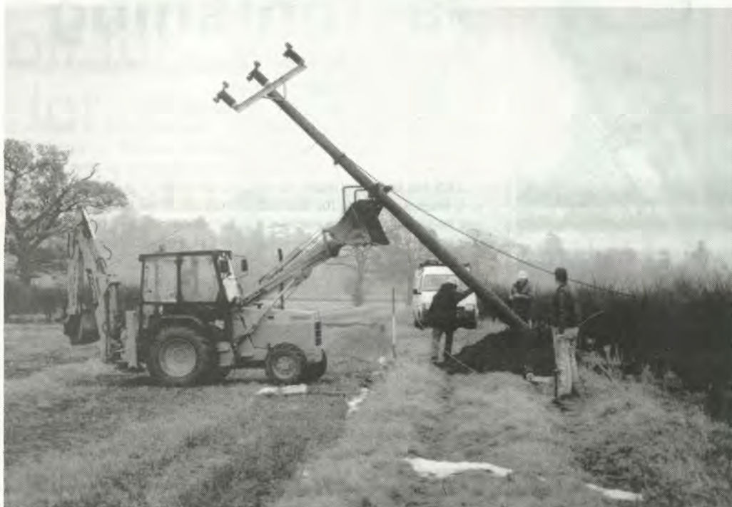
Wooden poles snapped like matchsticks in the high winds. Members of the Clwyd contingent are pictured erecting a new pole with the help of a mechanical digger.
